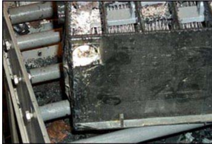
Corrosion --The positive terminal of this battery corroded so badly it became fused to the cable and broke. Note the internal corrosion on the strap and plates.
