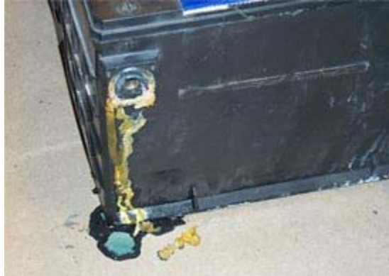
Battery Condition - This battery is leaking from a loose positive post and should not be tested. The battery is finished.
